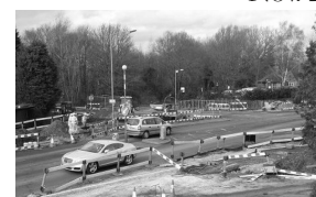
Bisley Roundabout under construction 2007
